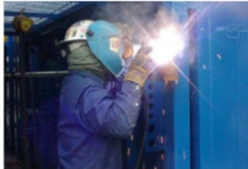
Figure 3: Welding - Hot work.
